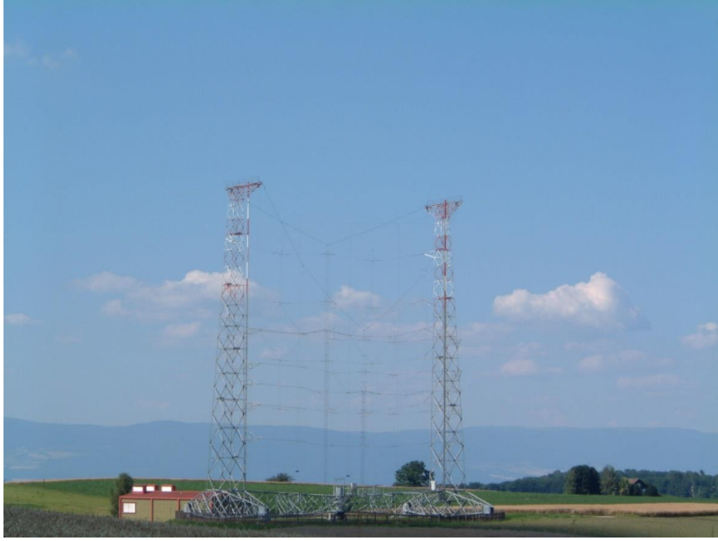
Short wave radio transmitter station – Example can be seen at KBC Langata and Ngong Radio transmission stations.
